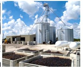
Florida (drying facility)
